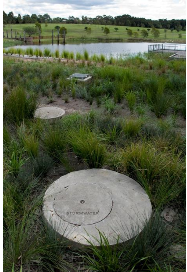
Sydney Park wetlands - stormwater
